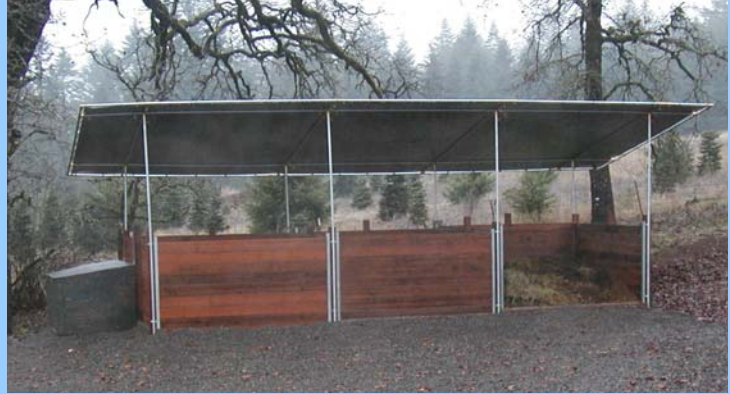
Three-bin manure composting system in use
