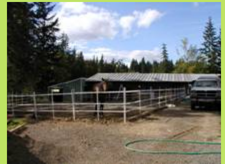
Heavy use protection area project complete
