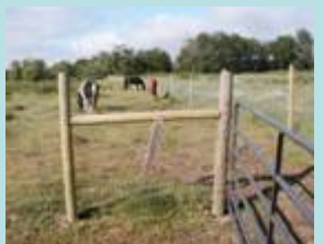
Completed fencing project
