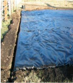
Geotextile fabric installed on bare ground and tucked into trench
