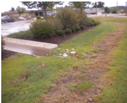
It is beneficial to deliver drainage water from a parking lot to a creek by first draining it through a bioswale before it is discharged, with riprap at the outfall of the discharge.
