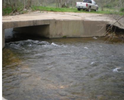
Low-water bridges installed without proper design can often block or limit both water flow and aquatic life movement up and down stream.
