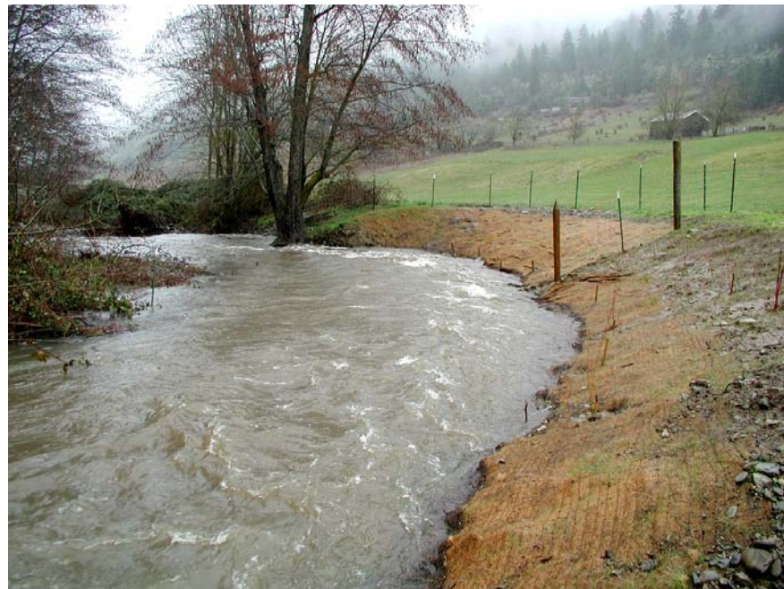
Figure 15. Erosion-control matting was used on this section of Thompson Creek in Jackson County, Oregon, after a steep, eroding bank was graded back to a more desirable angle, exposing bare soil. The site was revegetated with willow cuttings (visible as stakes in the fabric) and grass.
