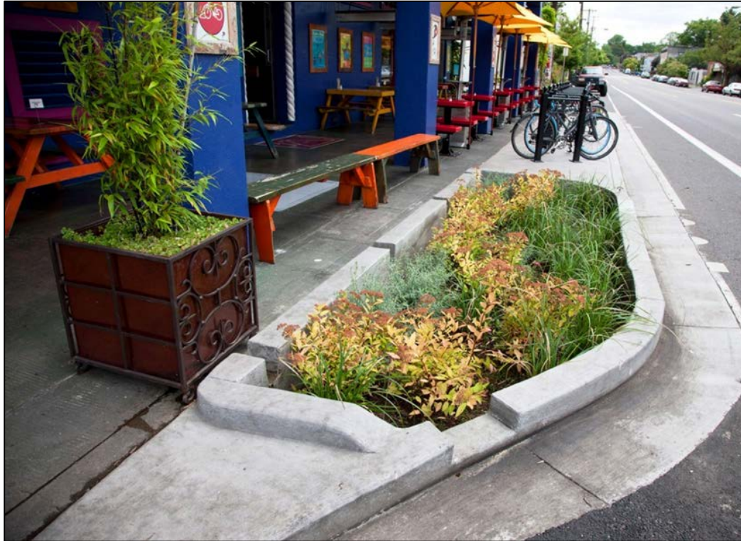
Curb extensions are street-side landscape areas which store, filter, and infiltrate stormwater runoff. Photo credit: Henry Ngan.
