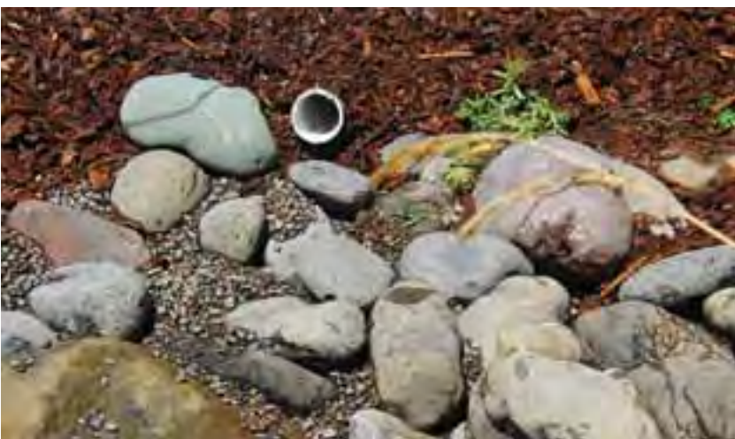
Figure 16: PVC pipe outflow from a coastal Oregon rain garden. The rocks, mulch, and gravel help protect the area from erosion. (Photo: Robert Emanuel, OSU)
